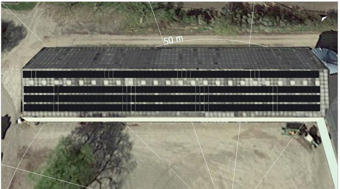
Illustration: 2. Modulflade - Building 01-Roof Area East
